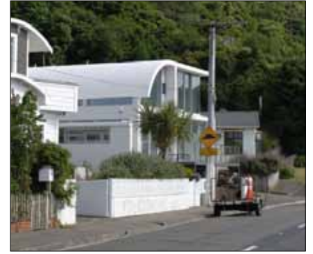
As Built View
